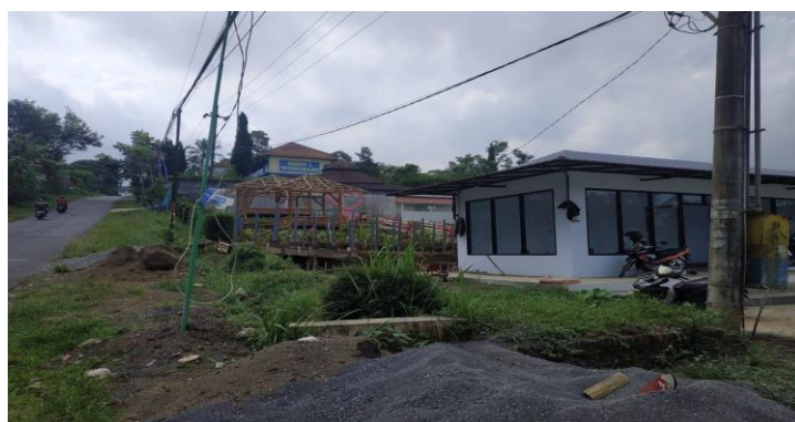
Figure 12. Rest Area Front Yard Construction
